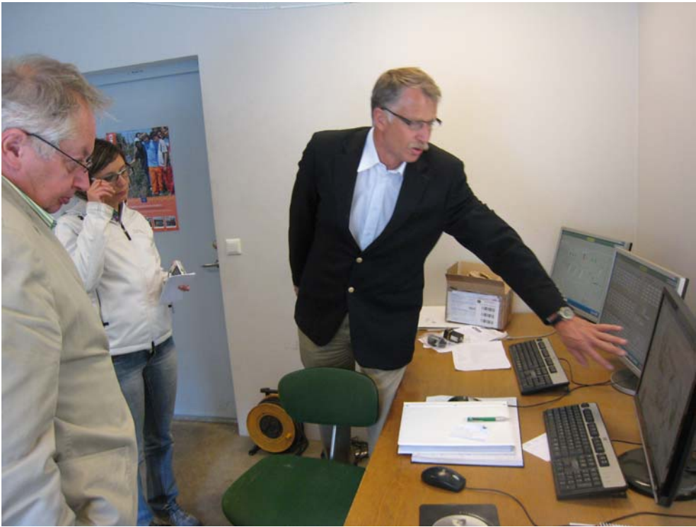
...and showing the control system for the automation of the BIOAGRO facility.
