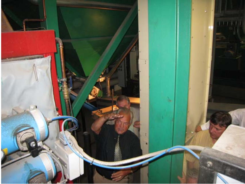
Gert Tarstad showing the 250 kW BioBoiler from HOTAB.
